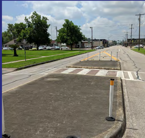
Mid-block crossing and pedestrian "refuge", one of many designs used to slow down traffic and promote pedestrian safety.
